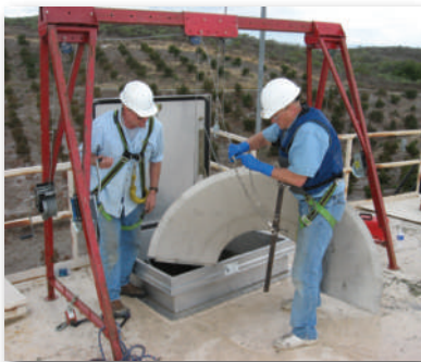
Installation Through Hatch
