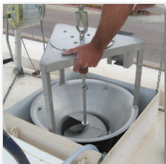
Installation Through Hatch
